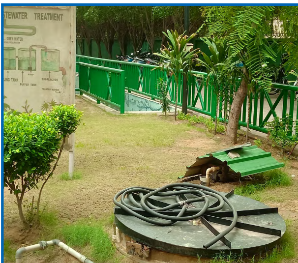
Waste water treatment plant at campus
